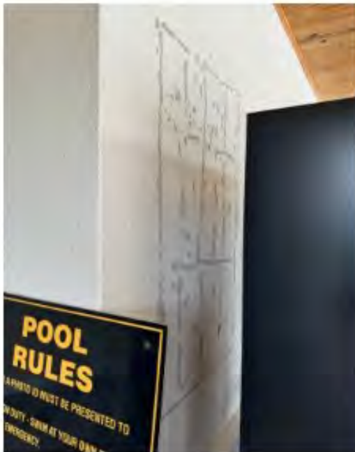
Repair damage area (stucco)
